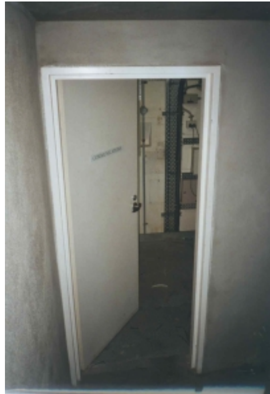
Sufficient access should be provided into riser shafts
