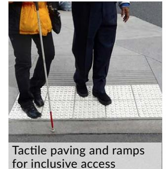
Tactile paving and ramps for inclusive access
