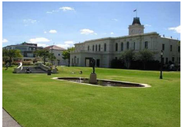
Figure 7: Vista through Town Hall Gardens to former Town Hall and former Khyat's Hotel. Note pond and statue.
