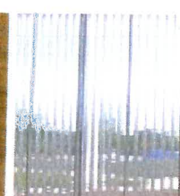
EF-05 TRANSLUCENT POLYCARBONATE WITH TIMBER BATTENS BEHIND
