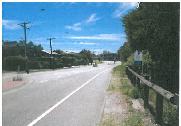
Two lane road with exclusive bicycle lanes near Deauville Street 12
