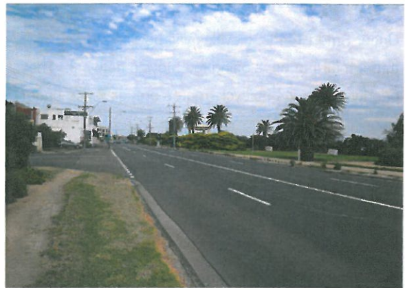
Four lane undivided road along Beach Road through Sandringham
