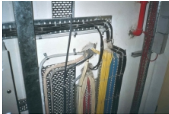
Wall penetrations re-instated and fire rated
