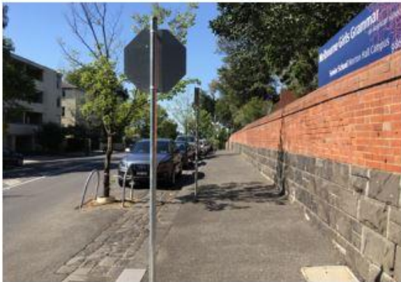
Original condition as a bitumen footpath (April 2017).
