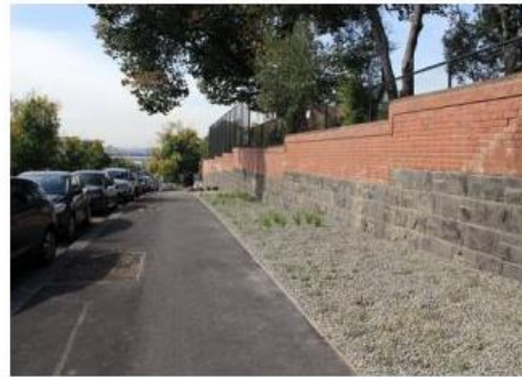
Plant installation (April 2018).
