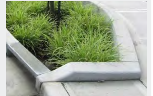
Formed concrete edges
