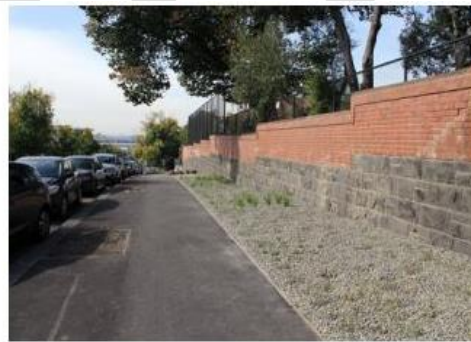
Plant installation (April 2018).
