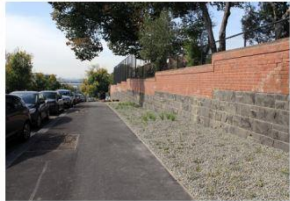
Plant installation (April 2018).
