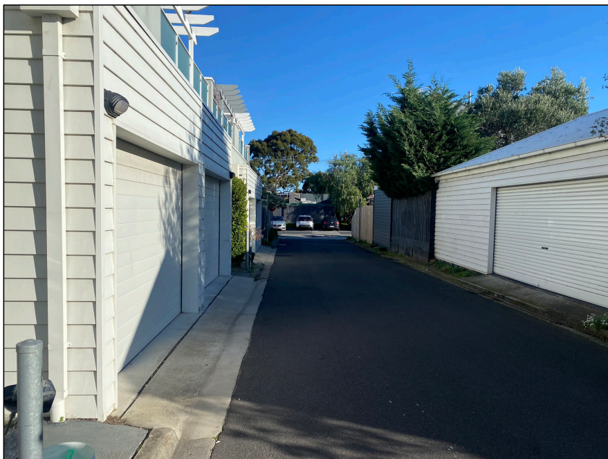
Figure 24 Garage restricted sight lines
