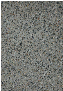
CON-03 DRIVEWAY - EXPOSED AGGREGATE CONCRETE
