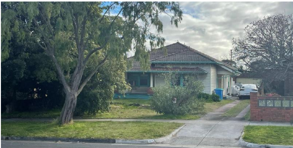
Figure 4: view towards the adjoining property to the west (115 Wickham Road)
