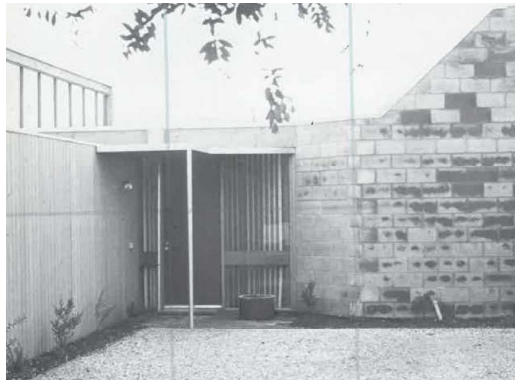
Figure 20: Coakley House, 4 The Avenue, Hampton (Source: N Day, Modern Houses Melbourne, p 164).
