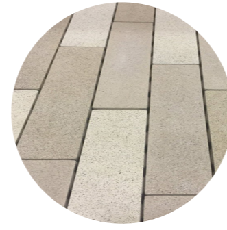
Exposed Aggregate Pre-cast Concrete Pavers
