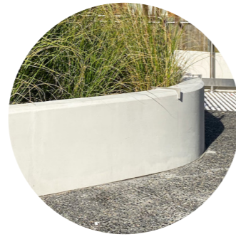
In-situ Concrete Seating Wall
