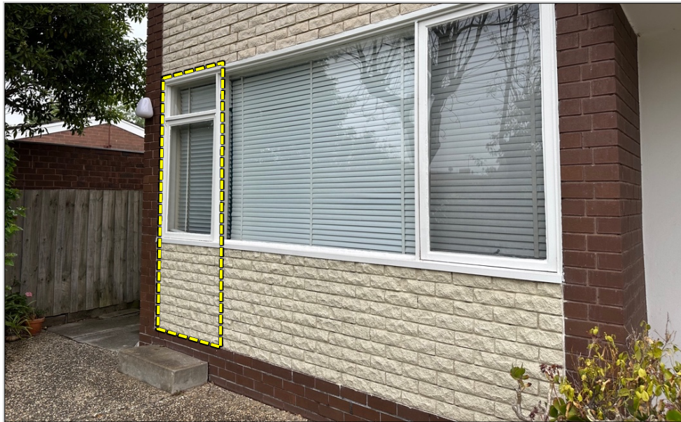
Figure 7 Part of the north elevation showing the location of an original door opening, replaced by brick infill and a window. Note the concrete step to the doorway has been retained.
