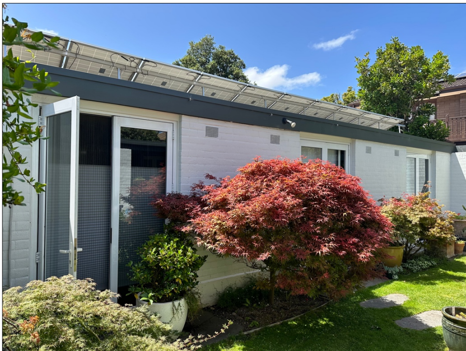
Figure 7 The southern external wall to the courtyard, as seen now. The face brick seen in the above image is now bagged and painted, the former timber doors replaced with aluminium framed doors and the courtyard has been re-landscaped (subsequent to the insertion and then removal of a swimming pool). The solar panels that have been added to the roof detract from its original rectilinear character.
