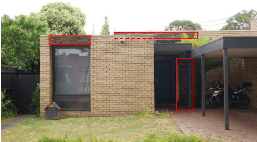
Figure 7. 19 Haywood Street - detail showing locations of stacked stone veneer finish (indicated)
