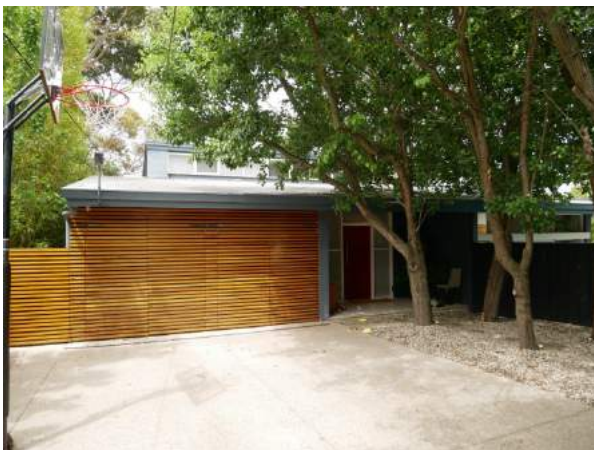
Figure 3. Eastern part of the street (north) elevation, 56 Cloris Avenue (Source: GJM Heritage, November 2023).
