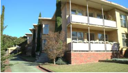
1-6/16 Clive Street, Brighton East (1960)
