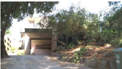
491 Balcombe Road, Beaumaris (VHR H2379 & HO412)
