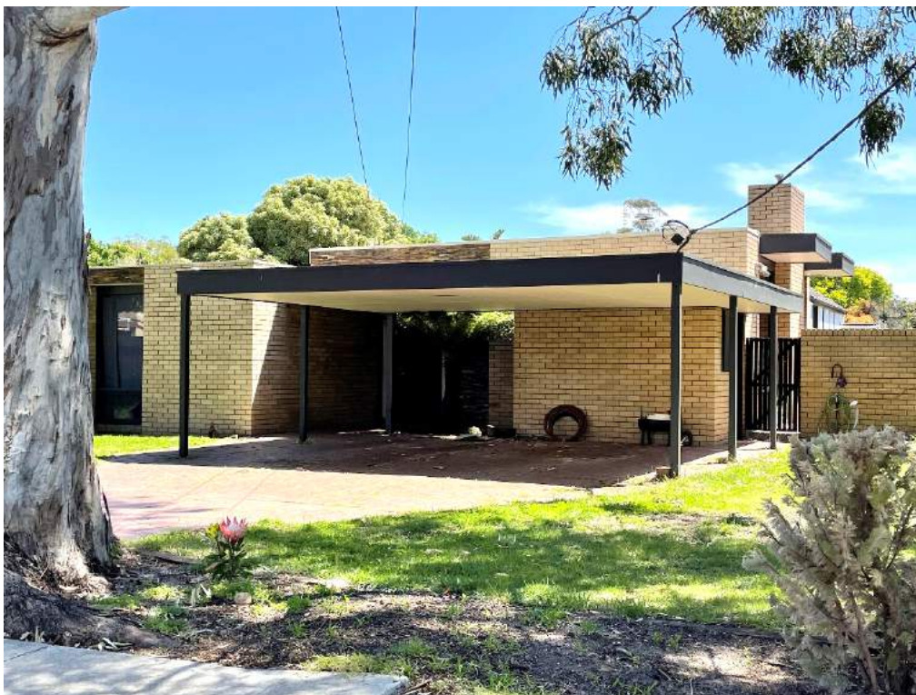
Figure 6. Carport and recessed entry (GJM Heritage, November 2021)
