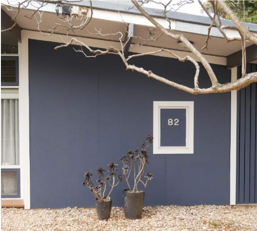
Figure 12. Detail of fibre cement sheeting, which has an applied textured finish
