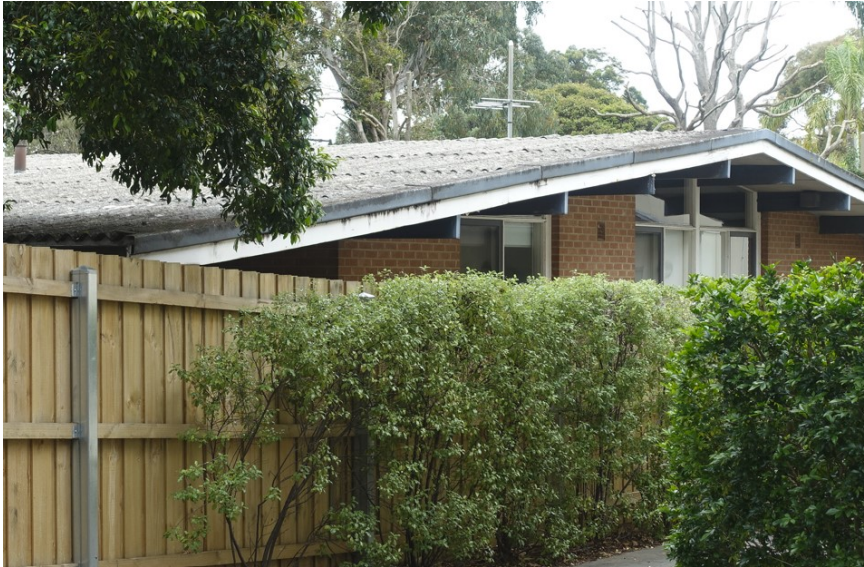
Figure 6. Rear elevation, as partially visible from Reserve Road, Dec. 2023. (N Schmeder)
