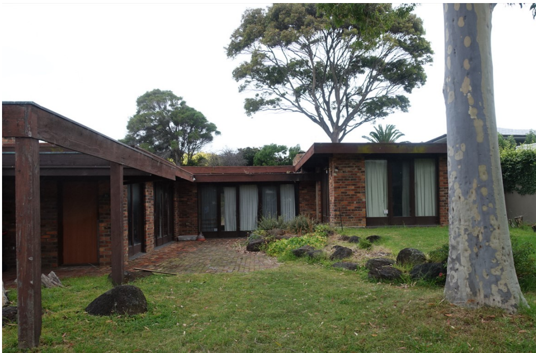
Figure 16. Front façade and garden of 21 Dudley Street, Feb. 2024. (N Schmeder)
