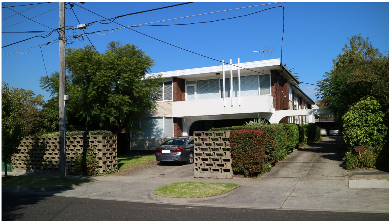
Figure 1. 16 Gillard Street, Brighton East (April 2021)
