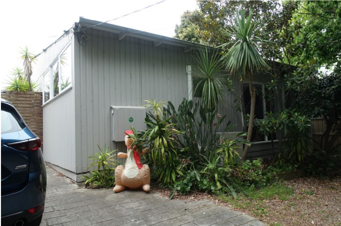
Figure 8. Front and part of the north side elevation of 78 Scott Street, Dec. 2023. (N Schmeder)
