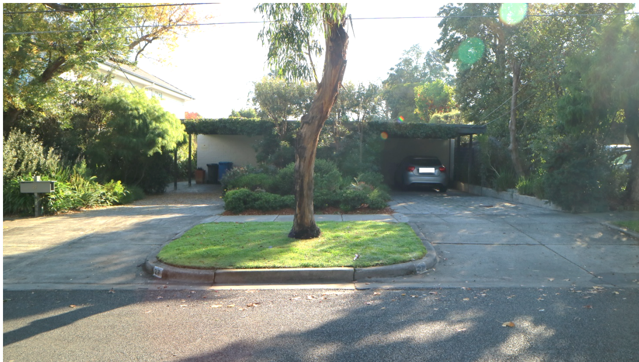
Figure 1. 27 Bolton Avenue, Hampton (April 2021)
