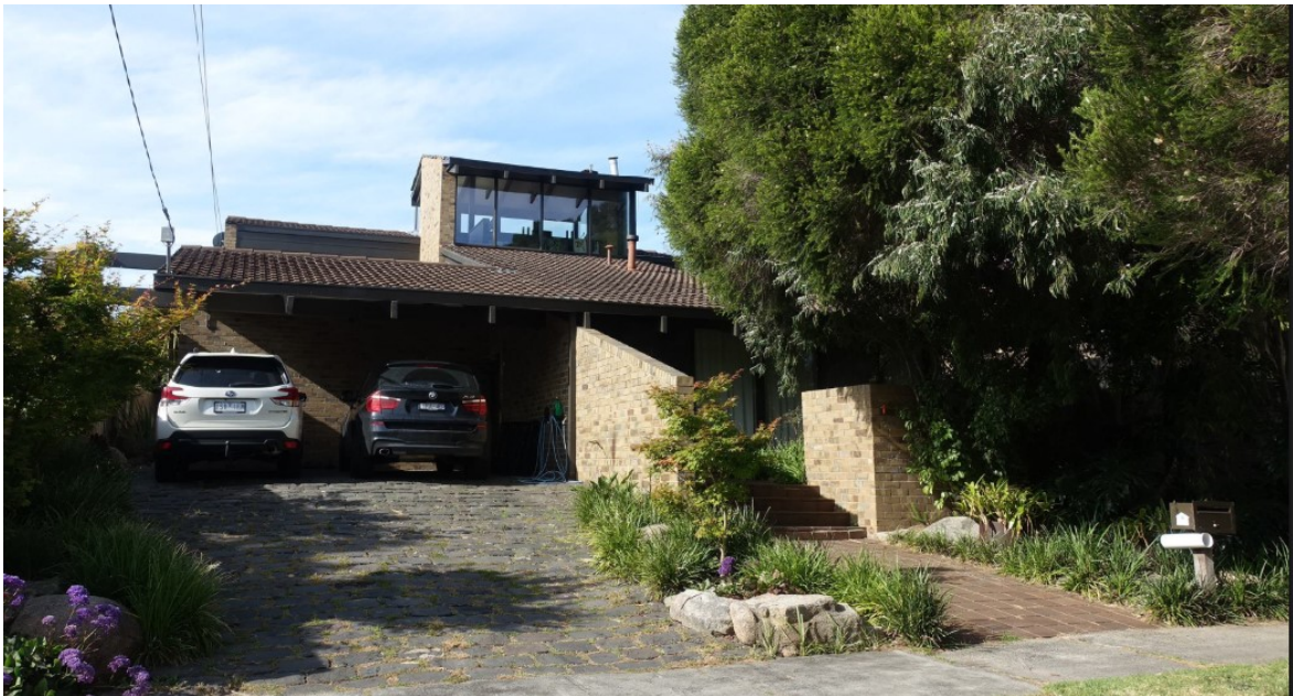
Figure 12. 1 Reid Street, Beaumaris, Dec. 2023. (N Schmeder)
