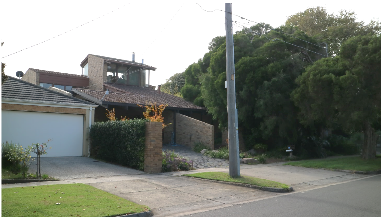
Figure 1. 1 Reid Street, Beaumaris (April 2021)
