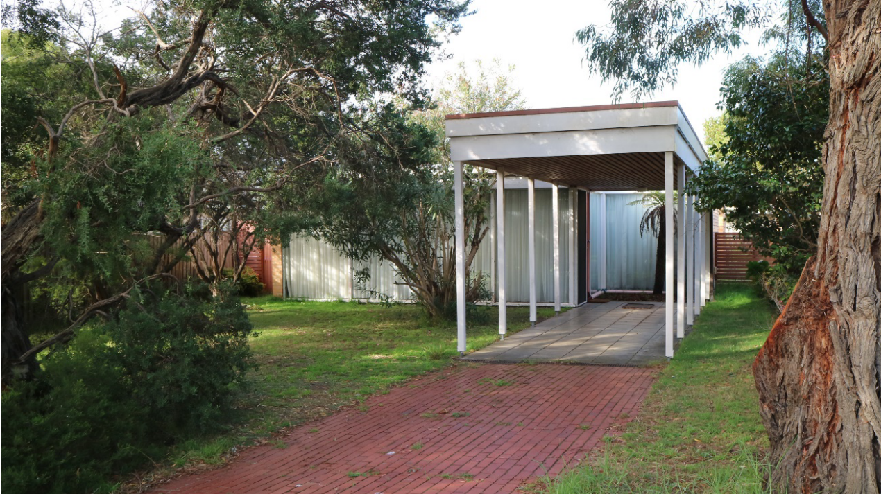
Figure 1. 28 Towers Street, Beaumaris (April 2021)
