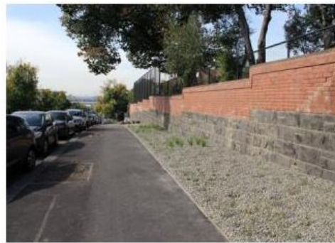
Plant installation (April 2018).
