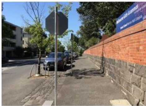
Original condition as a bitumen footpath (April 2017).
