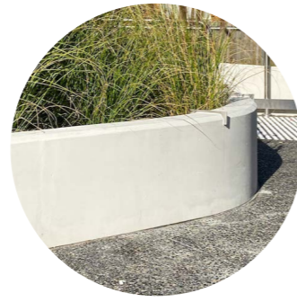
In situ Concrete Seating Wall
